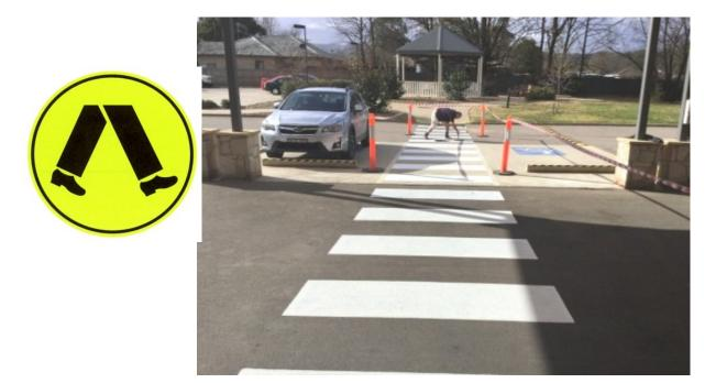
Pictured is John Carter from our maintenance department painting the lines, we have also erected a pedestrian crossing sign as a further reminder to us all to;
